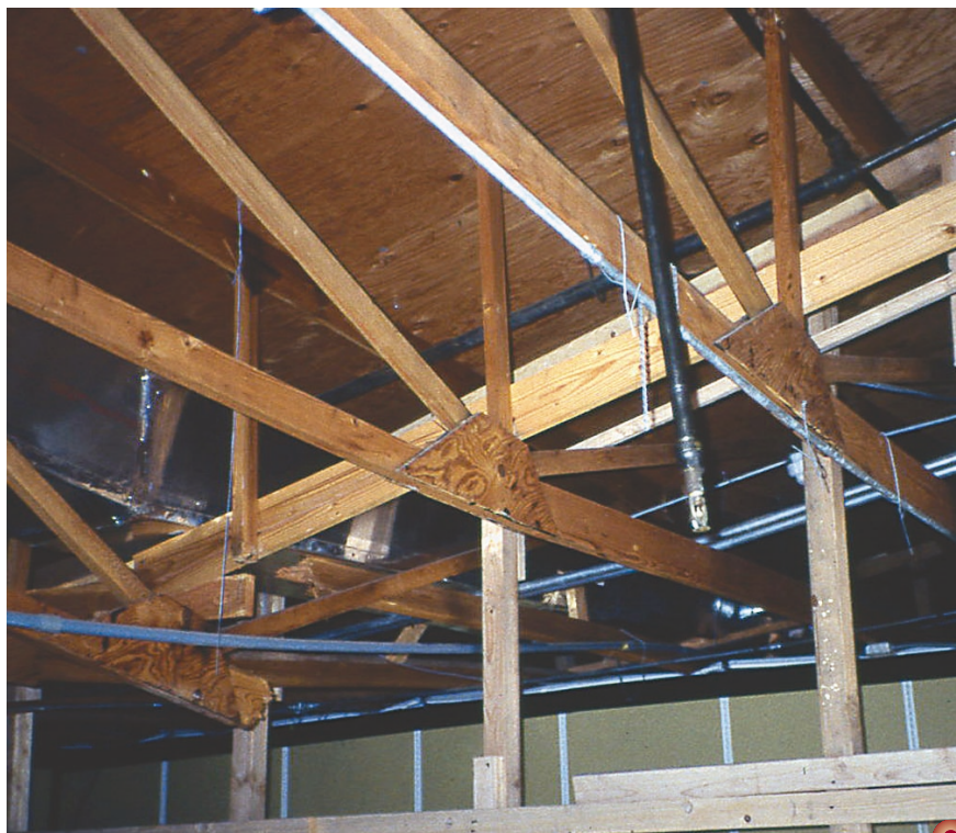
Trusses make it possible for buildings made of light-weight construction materials to last for years.
